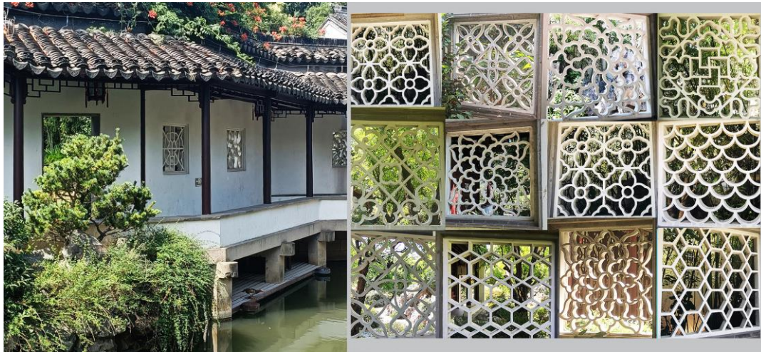
Figure 5 Single sided corridor and perforated windows in Zhanyuan (self-photography).
